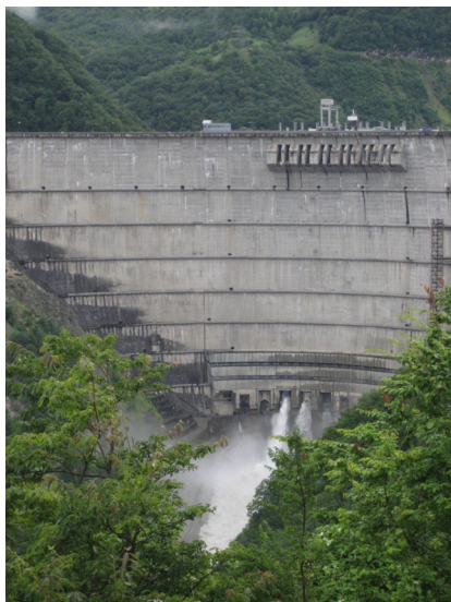
Figure 2: The dam of Enguri Hydropower Plant
