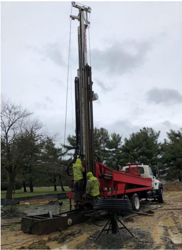
Figure 2 Geothermal drilling underway on property
