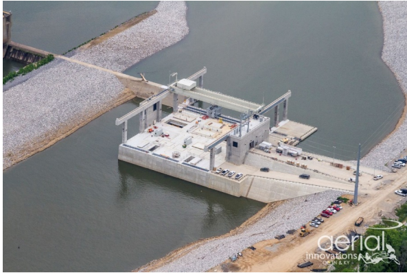
The 105-MW Meldahl Project at the Corps' Meldahl Lock & Dam
